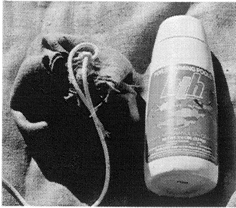
Fig. 1. Cloth sack filled with powdered chlorine compound is ready to be lowered into the well.
