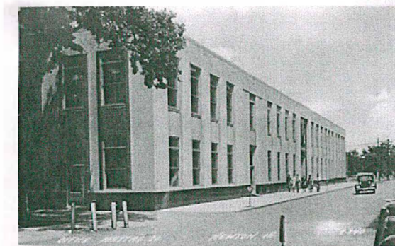
The 1935 Office Building was east of Bld. 1 and north of 4th Avenue (now the courtyard). It was not demolished when Building 20 (Headquarters) was built but rather encapsulated within the southwest part of the new Headquarters and the interior was remodeled to blend.
